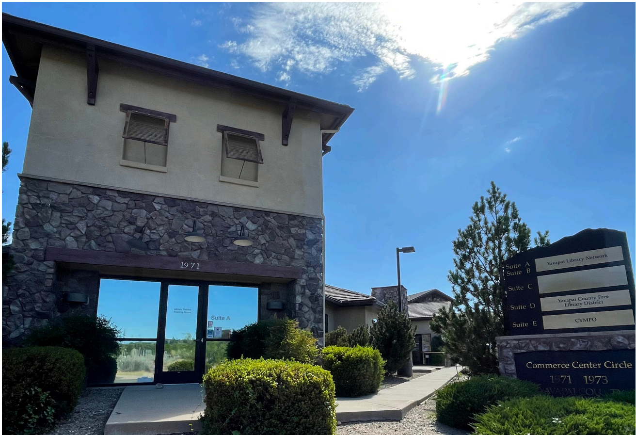
Yavapai Library Network and Yavapai County Free Library District Offices in Prescott, Arizona.
